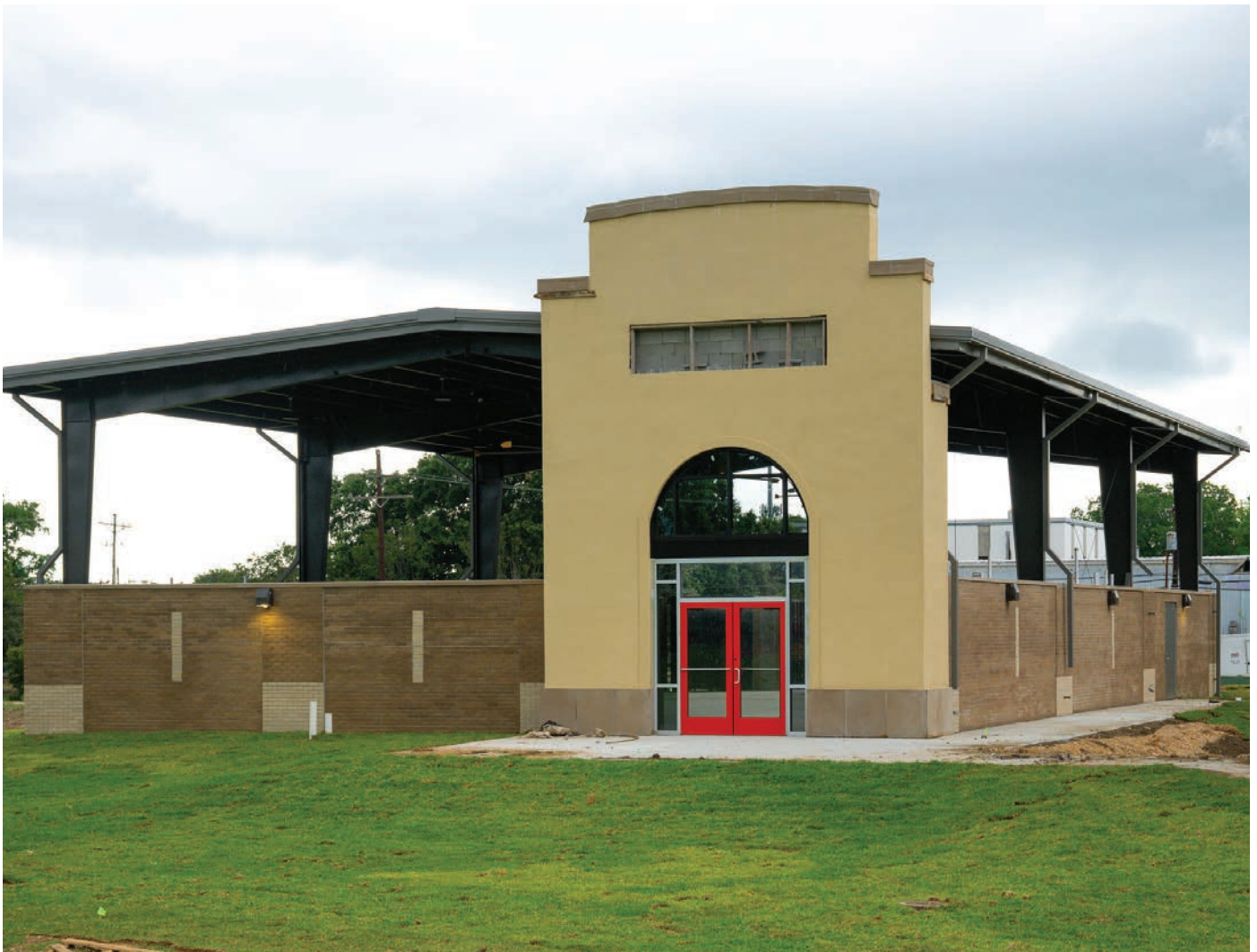
The Capital City Construction Lab is currently being built on the Mid City Campus, next to the Cypress Building.
